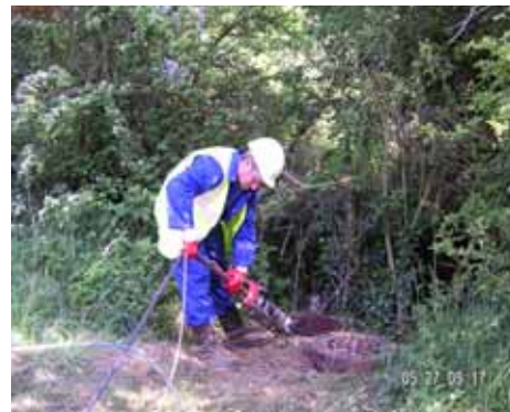
The Directional Root Cutter was placed by the manhole and attached to the winch rope ready to be placed in the pipe.
