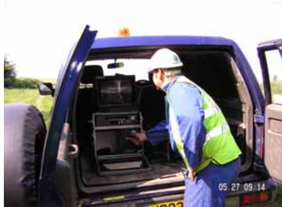
The operator was able to control and monitor the progress of the root cutting from the rear of a four x four vehicle.
